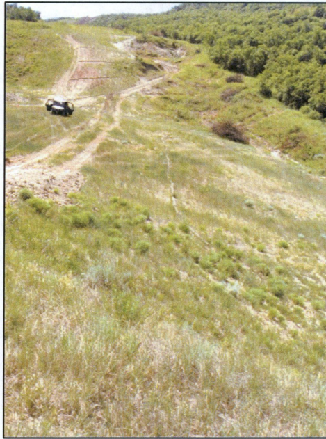
Photograph 7. View across regraded fill area along proposed DAPL centerline (marked by stakes). View to south.
